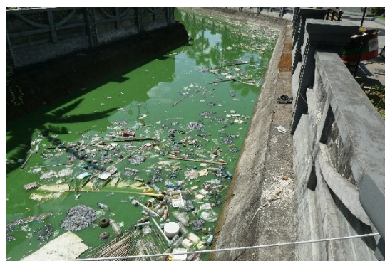
Still some problems with waste water
