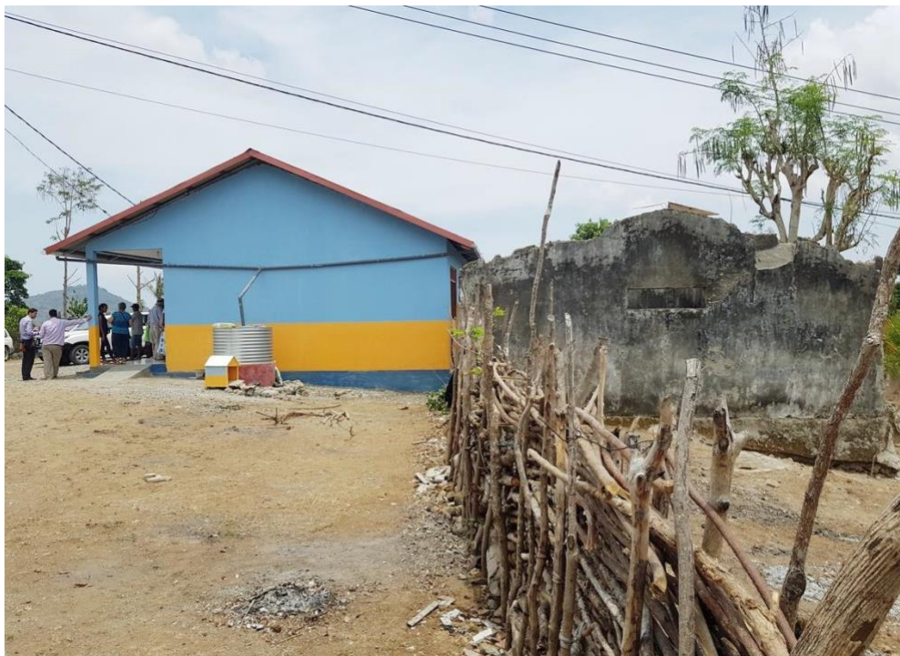
A school funded by Spend it Well (left) sits next to the building it replaced (right)
